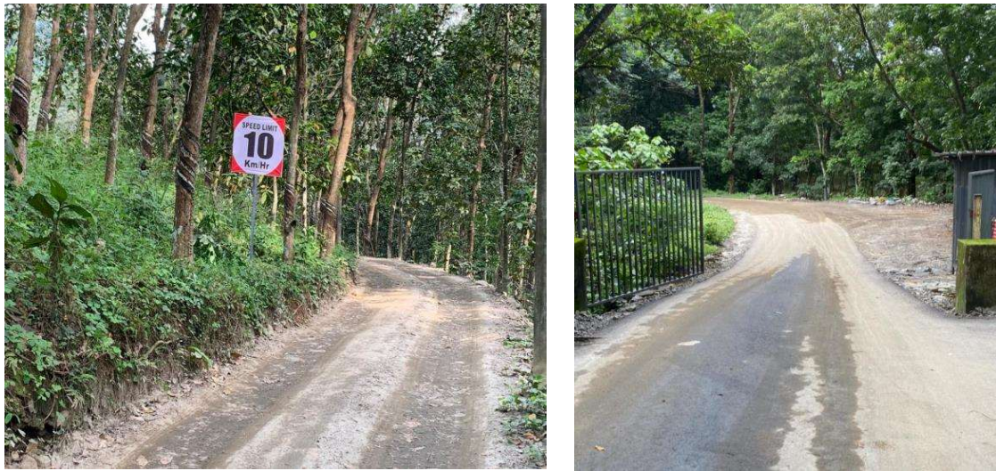
Figure 5: Photograph of Access Road to Quarry
